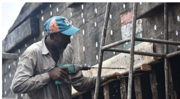
Fig. 1 Replacement of wooden plank in progress
