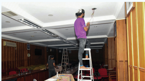
Replacement with energy efficient bulbs and lighting system in progress
